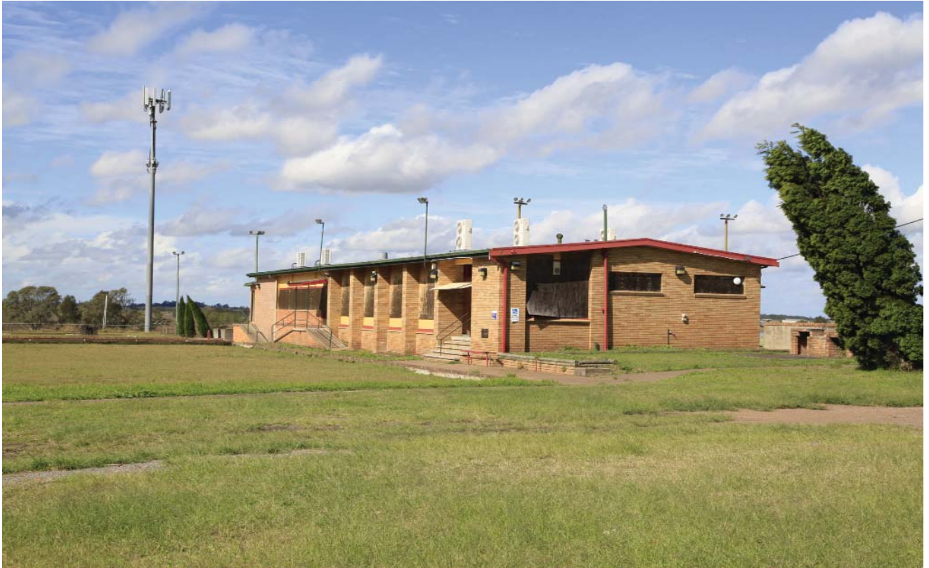
Location 9: Detail of former bowling clubhouse looking south east.
